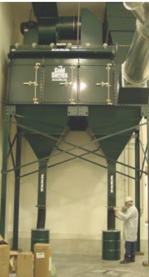
GS24 with top mount fan and vertical explosion vent
